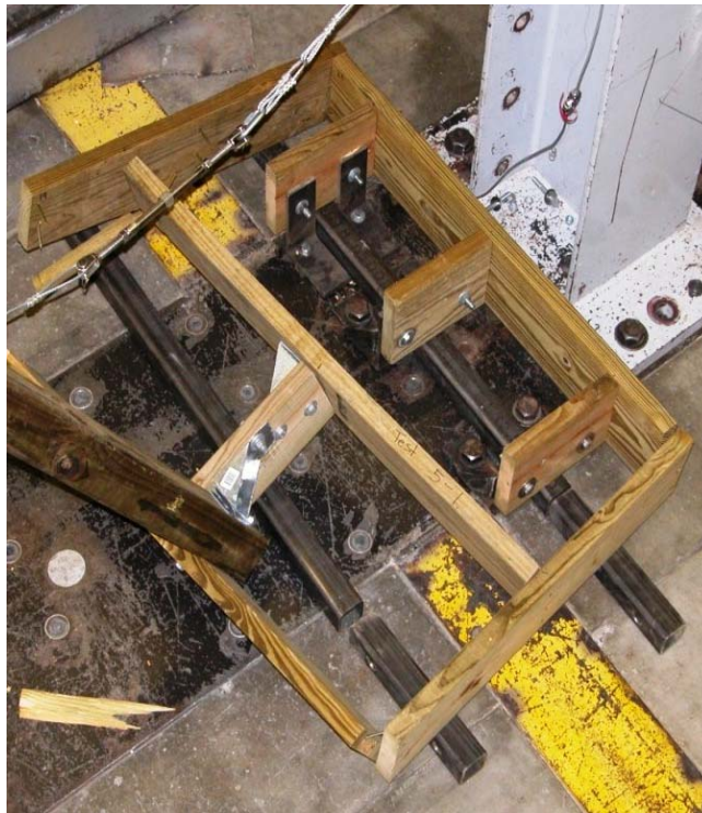
Figure A10. Failure mode for test specimen 1, configuration 5
