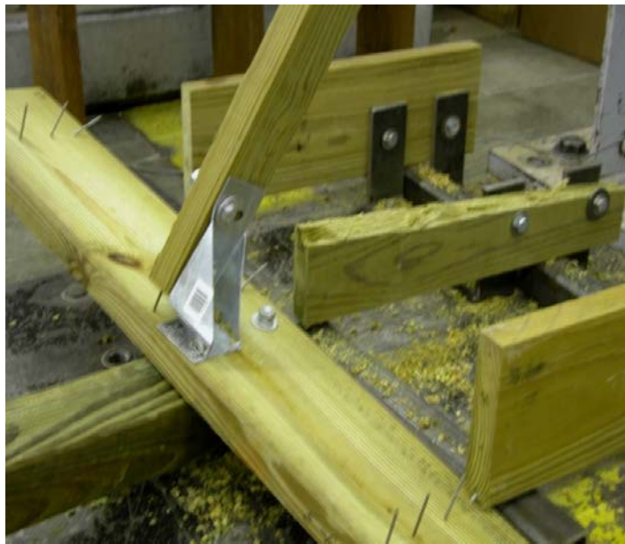
Figure A8. Failure mode for test specimen 3, configuration 3
