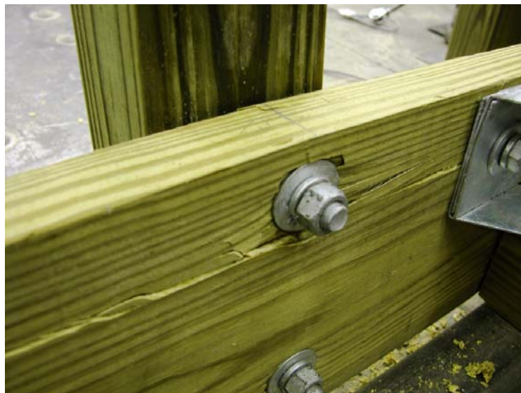
Figure A4. Failure mode for test specimen 3, configuration 1
