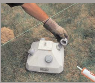
Make sure to remove any deformations on the end of the pin, and caulk and seal the cap.
