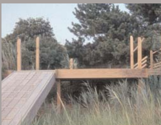
First deck on prototype pier - 1984 Lawrence, New York
