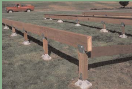
Frame Foundations for Modular Structures
