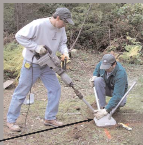
Hold pin up against the top side of the driving hole when driving.
